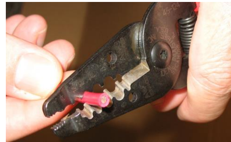
Figure 70. Strip 12 AWG Load Lead Wire
